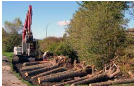
Big logs with roots attached cabled to big boulders guided by Gerry Oliver, RPBio
