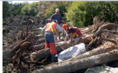
Big logs with roots attached cabled to big boulders guided by Gerry Oliver, RPBio
