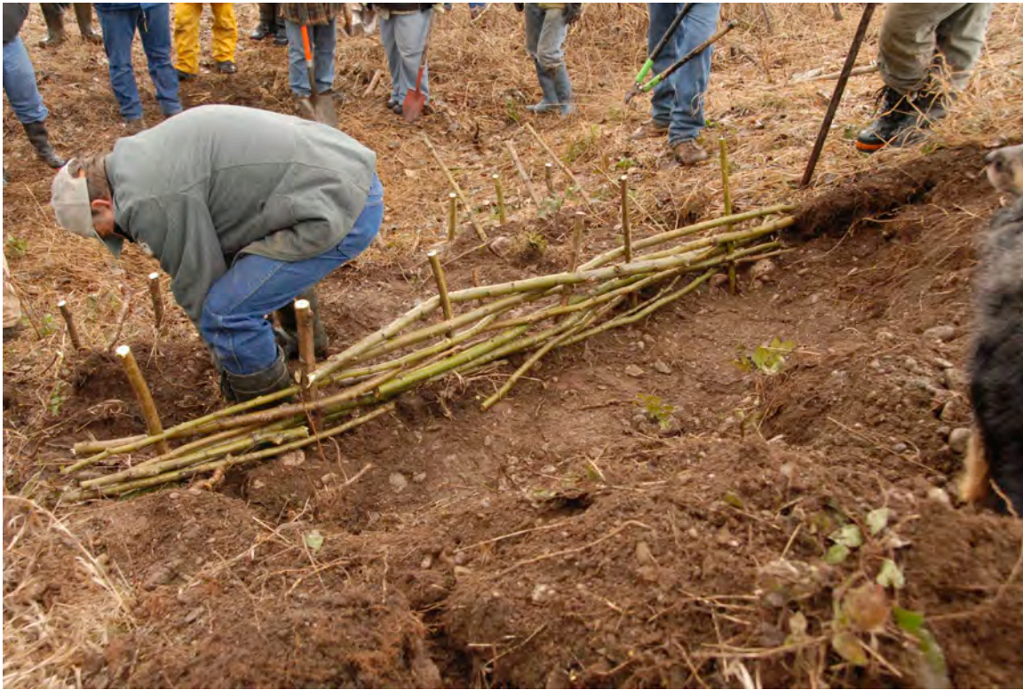
Constructing a wattle fence, which are also built with Cottonwood stakes
