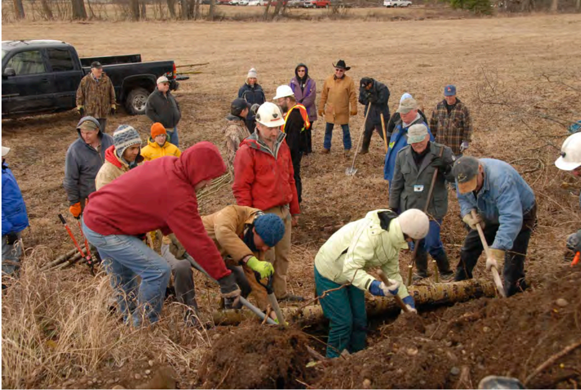
Constructing brush layers
